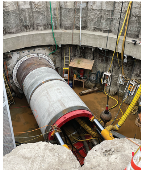
Installing the Integral IJS Pipe into pipe string
