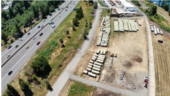
Open Cut FRP and Flow-Crete™ staging area
