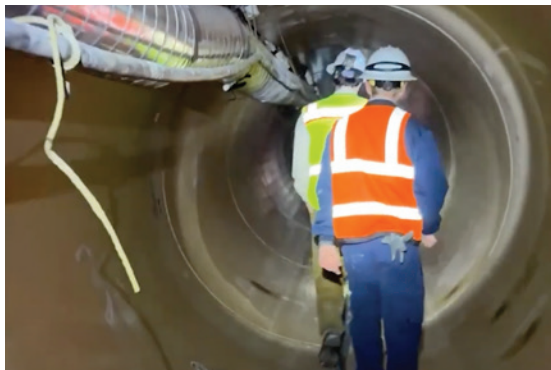
Final Inspection of installed pipe before flooding tunnel
