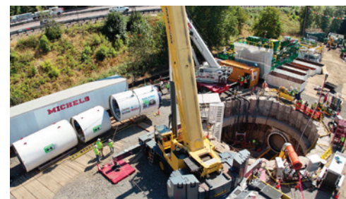
Lowering the MTBM named "Whack-A-Mole" lowered into launch shaft
