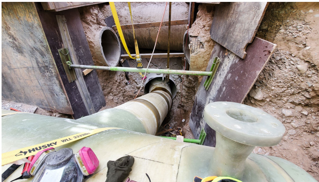
Figure 5. Tee intersection fitting and blow off of 36" to 30" FRP sewer force main.
