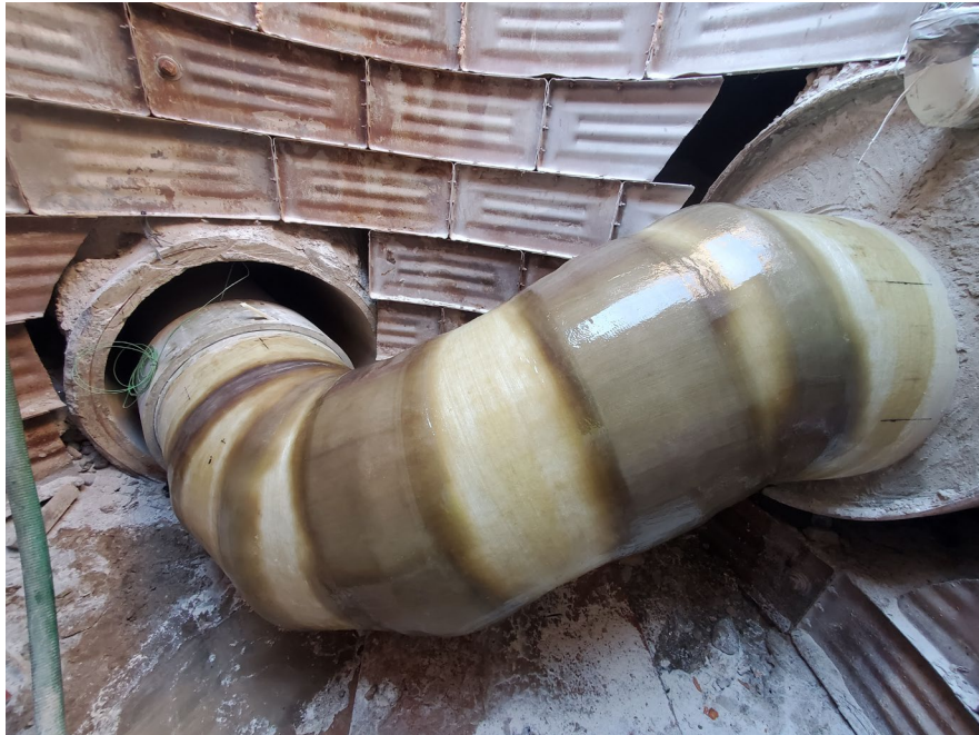
Figure 3. A custom fitting made on site at an access pit where 2 tunnels meet. Making fittings like these on site proved very useful in design build situations.
