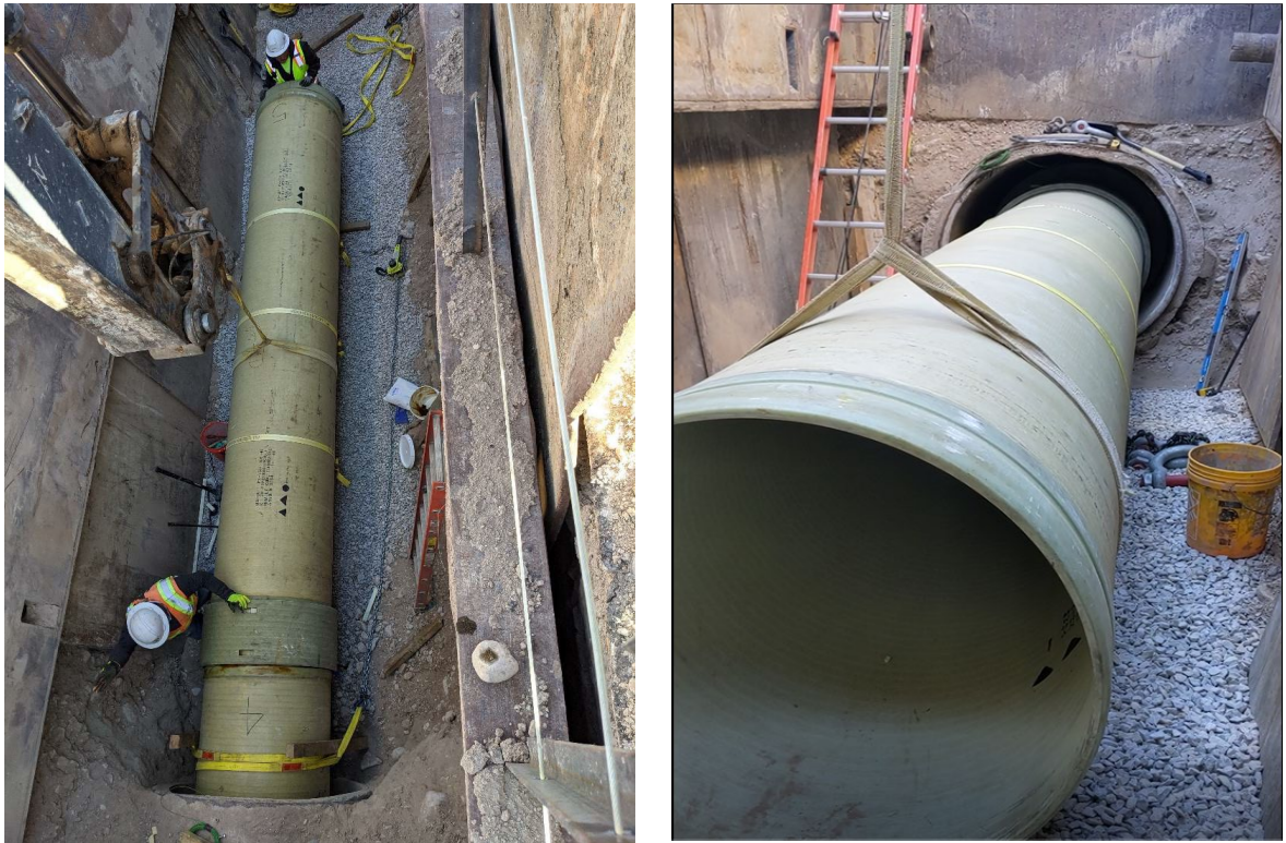
Figure 4. ORC performing FRP pipe slipline installation.
