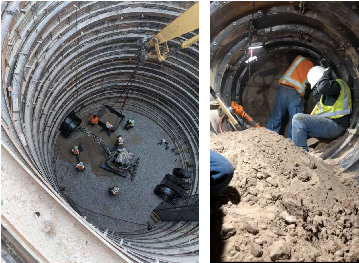
Figure 6. ORC hand tunneling operation. 30' diameter access pit on left. Hand tunneling shaft on right.
