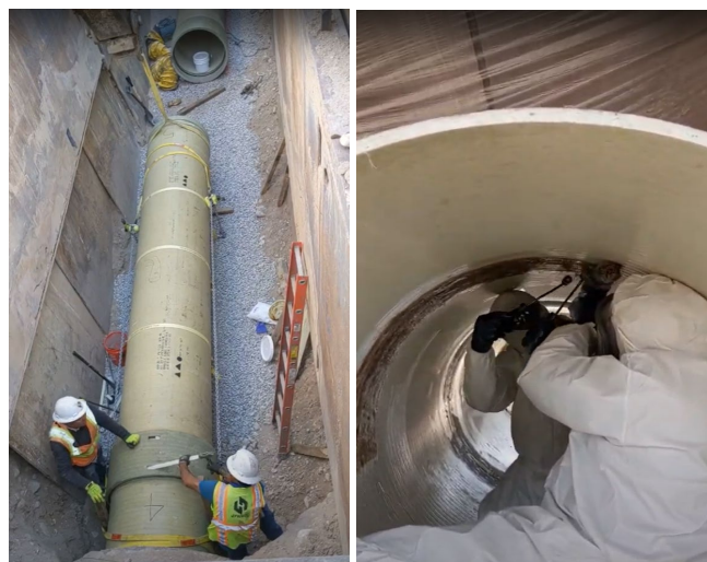
Figure 2. Two forms of restrained joints. Installation of a Key Lock with lock rod on the left. An internal butt wrap laminate joint on the right. Butt wraps can be performed both internally or externally.
