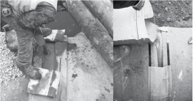
grout band attached to pipe with steel straps sewn into the hems
