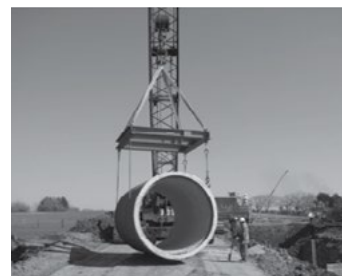
crane handling pipe using a lifting sling assembly
