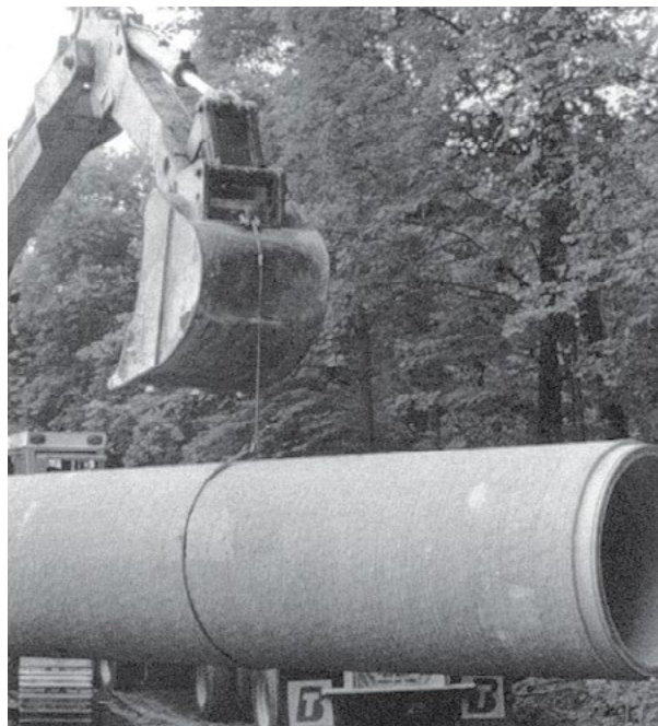
backhoe picking pipe up with sling
