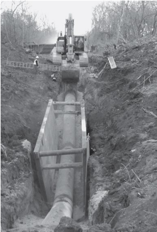
backhoe is used to backfill pipe
