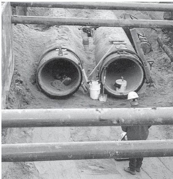
preparing the trench for the next pipe length
