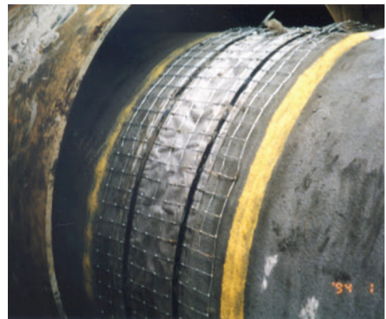
Figure 4: Light gauge steel mesh wrapped around the joint to support the wet grout in the grout band.
