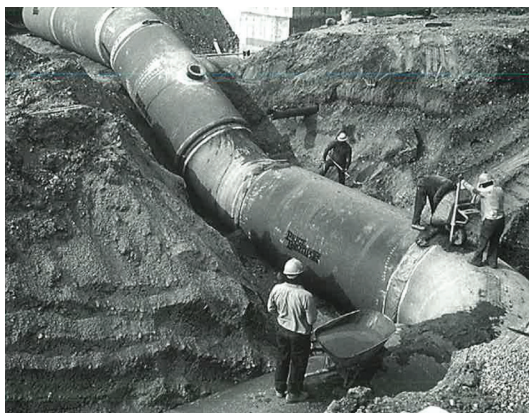
PCCP is ideally suited for many applications, such as this treatment plant. The precise custom fittings made this complex installation simpler to install with no field cutting or tapping.
