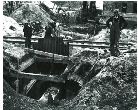
An early installation of prestressed concrete cylinder pipe.
