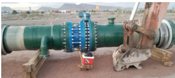
Flanges may be bolted to the pipe to hold joints together.
