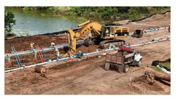
the hard rock below. As an added precaution, the team enclosed the pipe with a concrete cage for additional protection from outside impacts. Elsewhere, a variety of fittings and elbows accommodated elevation changes and small creeks to follow the existing line.
