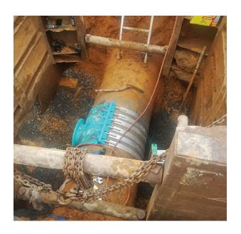
Research showed the city's 30" lined prestressed concrete cylinder pipe (AWWA L301) was put into service in the 1950s. An 8" hot tap helped expand service to a new facility.
