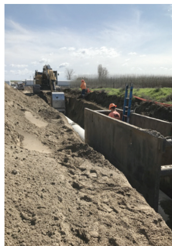
▲ PUSH ON JOINTS IN LENGTHS UP TO 40' ALLOW FOR FAST INSTALLATION. NO NEED TO PROTECT JOINTS AFTER INSTALL SINCE THEY ARE CORROSION RESISTANT.
