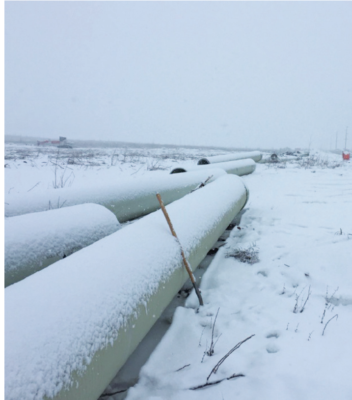
▲ FLOWTITE® FRP PIPE WITHSTANDS THE RIGORS OF SUB-ZERO WINTERS.
