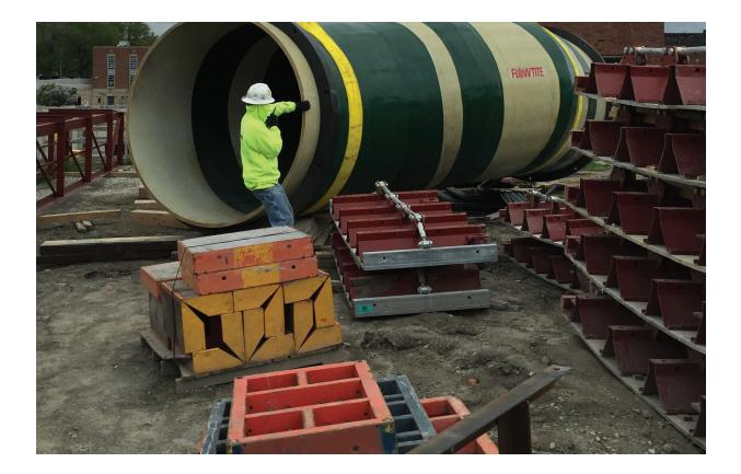
To address potential buoyancy issues, the pipe was anchored to a reinforced concrete slab wherever the 60-, 72- and 84-inch pipes were to be installed. This effectively eliminated any risk of buoyancy problems.
