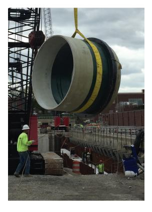
carbon fiber internal laminate restraints were used. Finally, for effluent conduits connected to rigid structures, bolted harness-style joints were used. This allowed the joints to maintain their flexibility.
