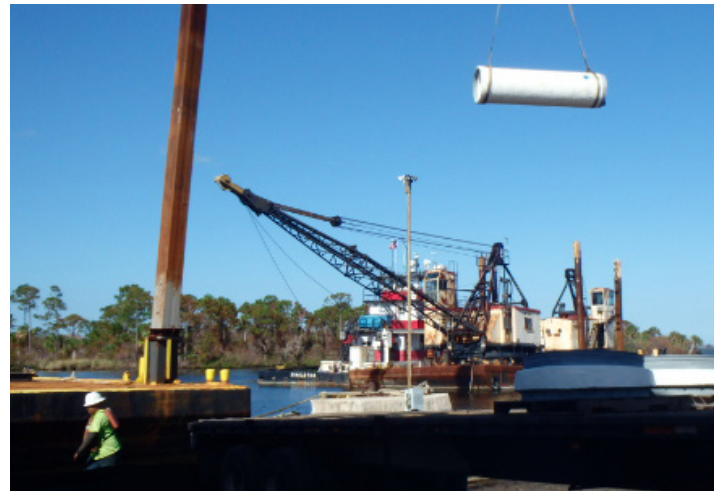
▲ SECTION OF 36" PCCP IS HOISTED INTO POSITION
