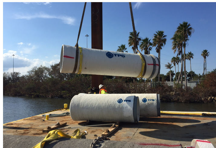
▲ BEVEL ADAPTER IS PRE-ASSEMBLED ON LENGTH OF PCCP
