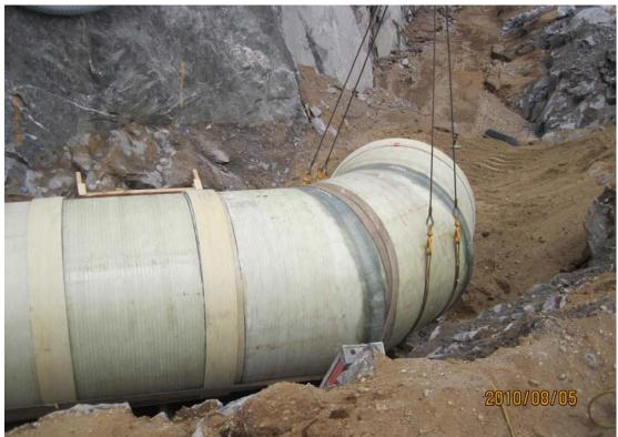
Figure 5 – 96 inch FRP Bend installation.
