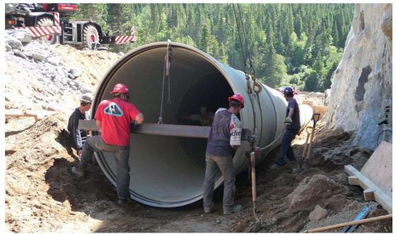
Figure 6 – Pipe section assembly using Come-a-longs and nylon slings.
