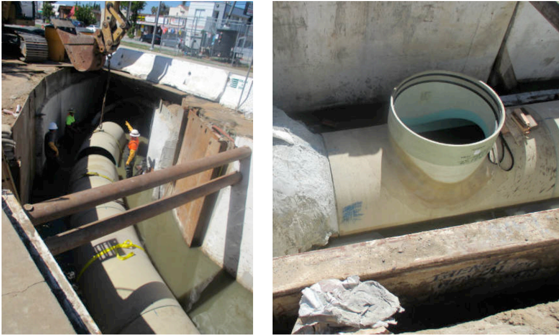
Figure 9: Installation Non-Round FRP Slipline Bend Segments and Manhole
