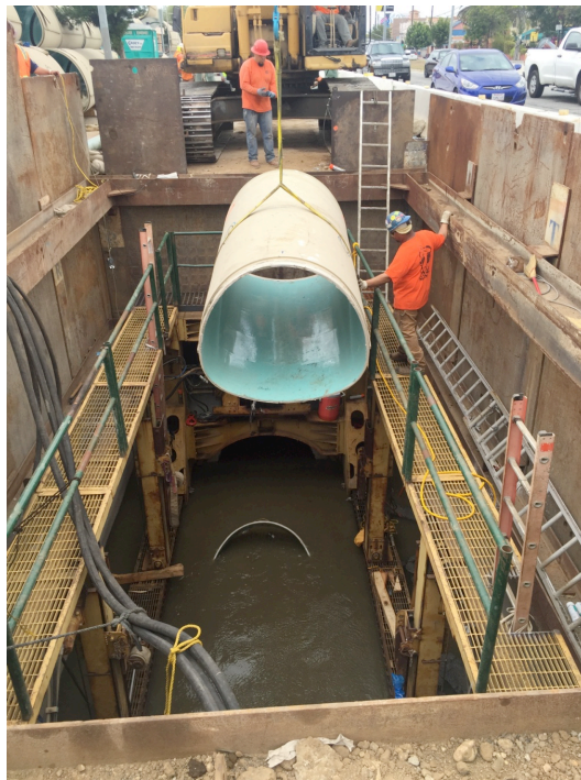
Figure 8: Installation of Non-Round FRP Slipline Segment
