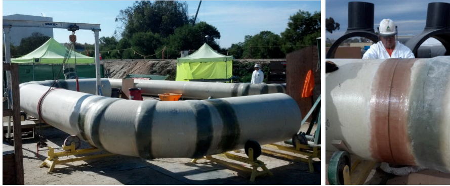
Image 2 – Fiberglass Field Laminations
