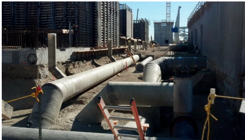
Image 1 – Fiberglass Pipe Installation
